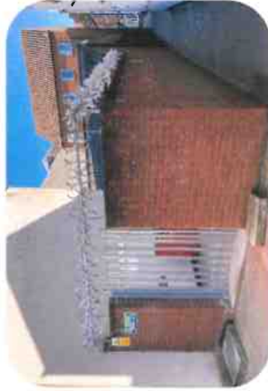
Rotating anti-climb spikes & gate, rear of The Halifax Bank, 15a The Cornmarket
